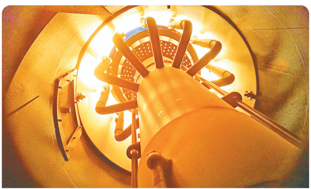
昨日,二马路“煤改气”项目点火成功
